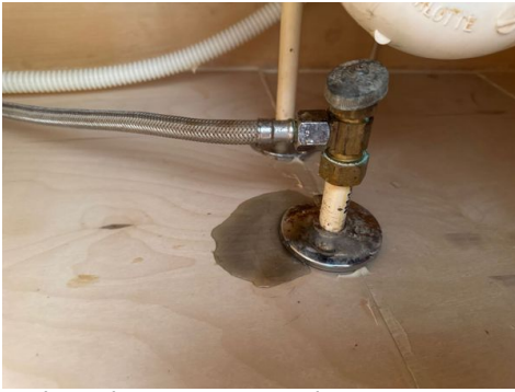
Dishwasher Water Supply Line
