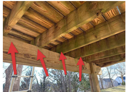
Missing Hurricane Straps
