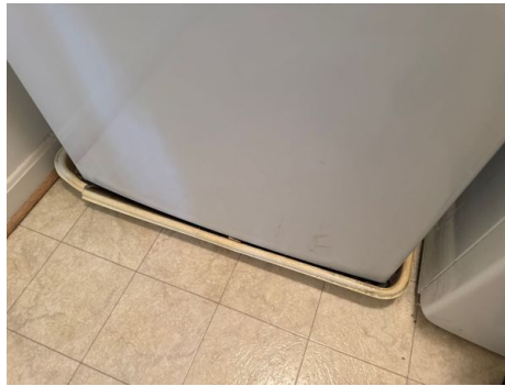
Washing Machine: Drain Pan
