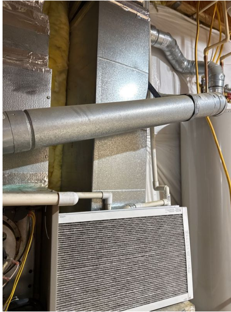
Heating Equipment : Flue Pipe Single Wall
